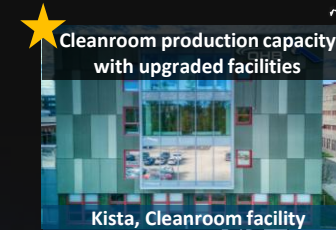
Kista, Cleanroom facility
